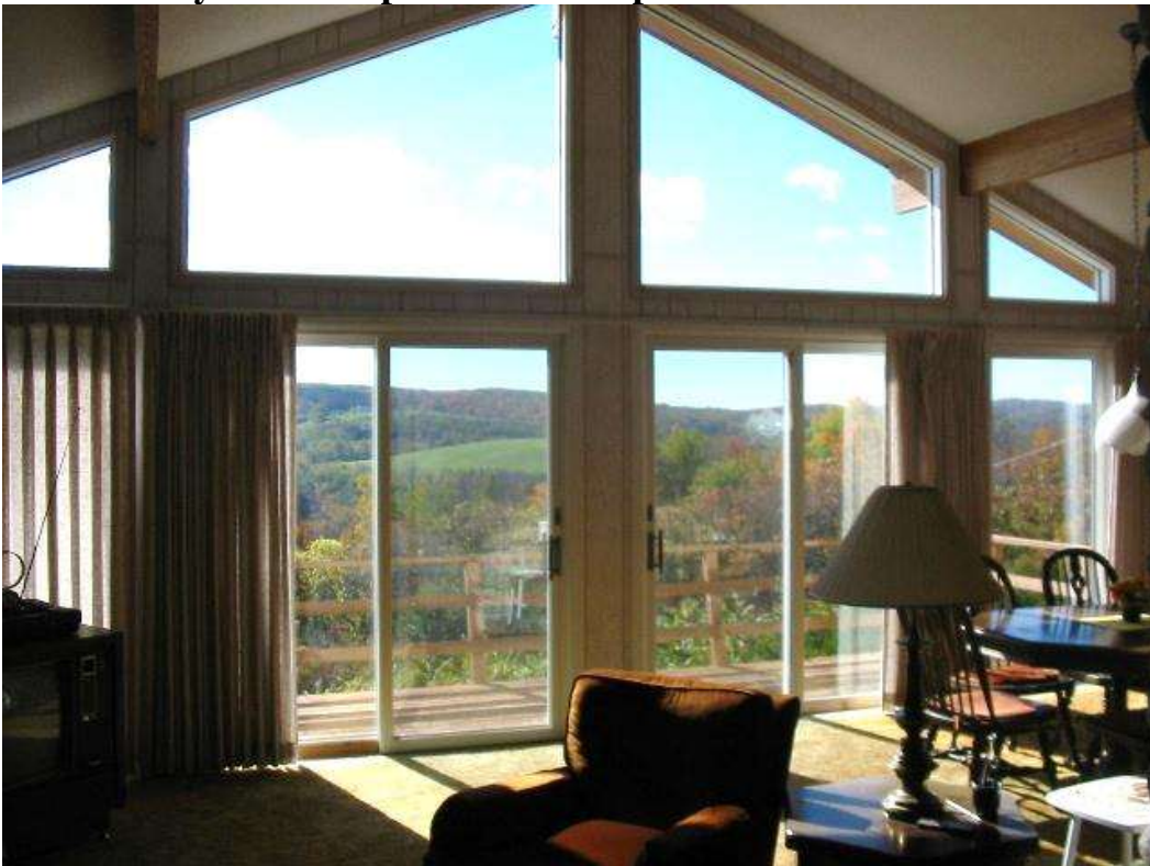
These heavy windows provide lots of passive solar heat in the winter
