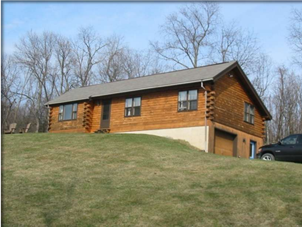
A real log home! Cute and cozy, with a full walk out basement and garage.
