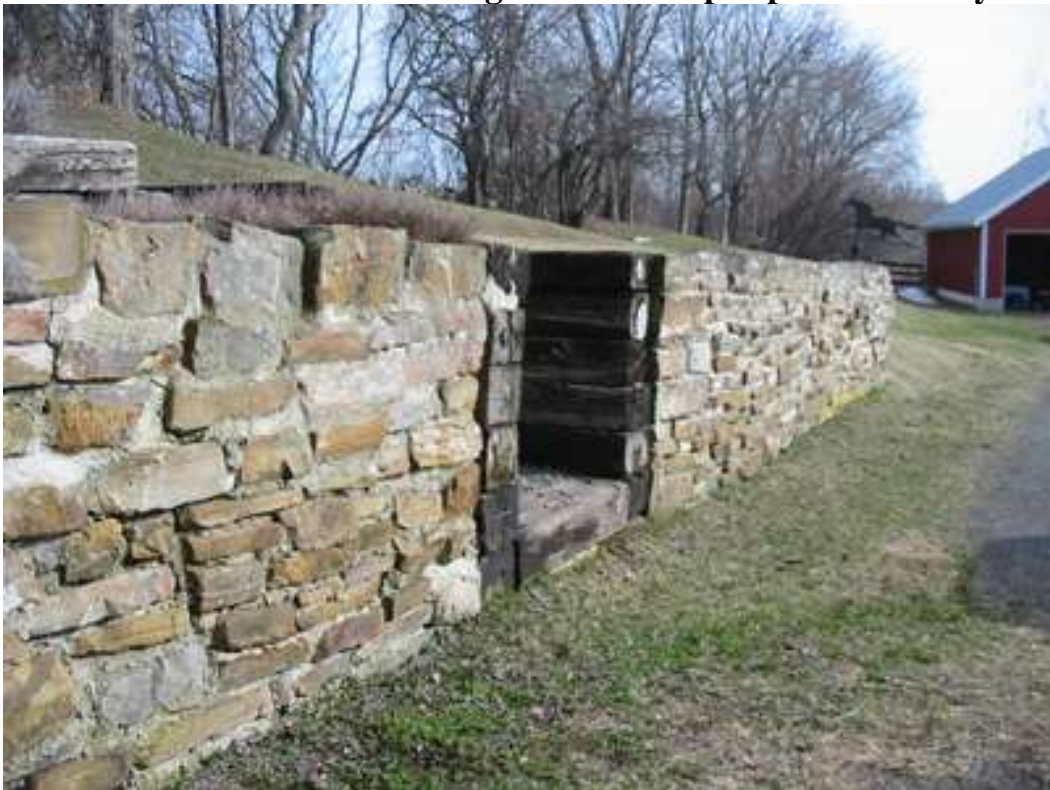
Beautiful natural stone retaining wall with steps up to the back yard.
