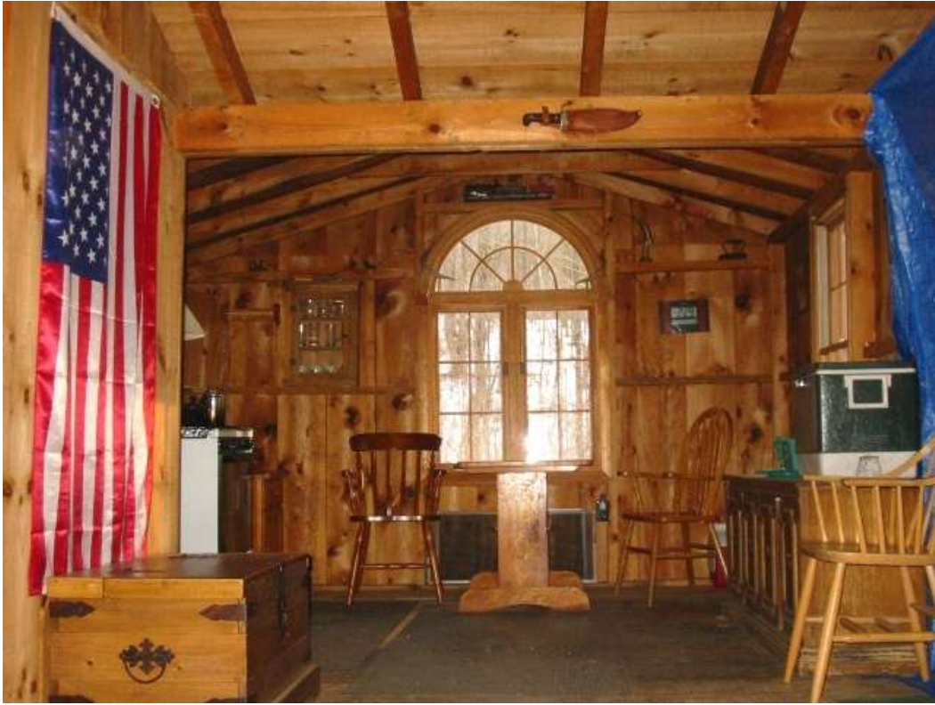
The interior is clad with rustic, natural rough sawn lumber.
