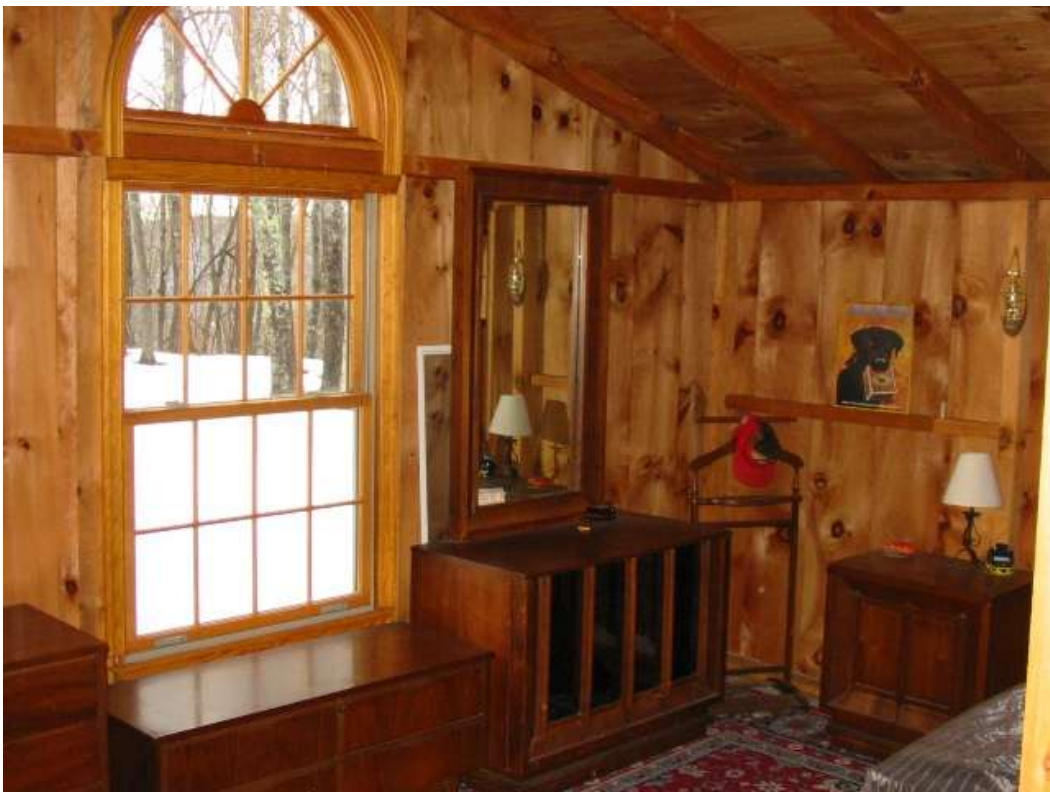
The interior is clad with rustic, natural rough sawn lumber.
